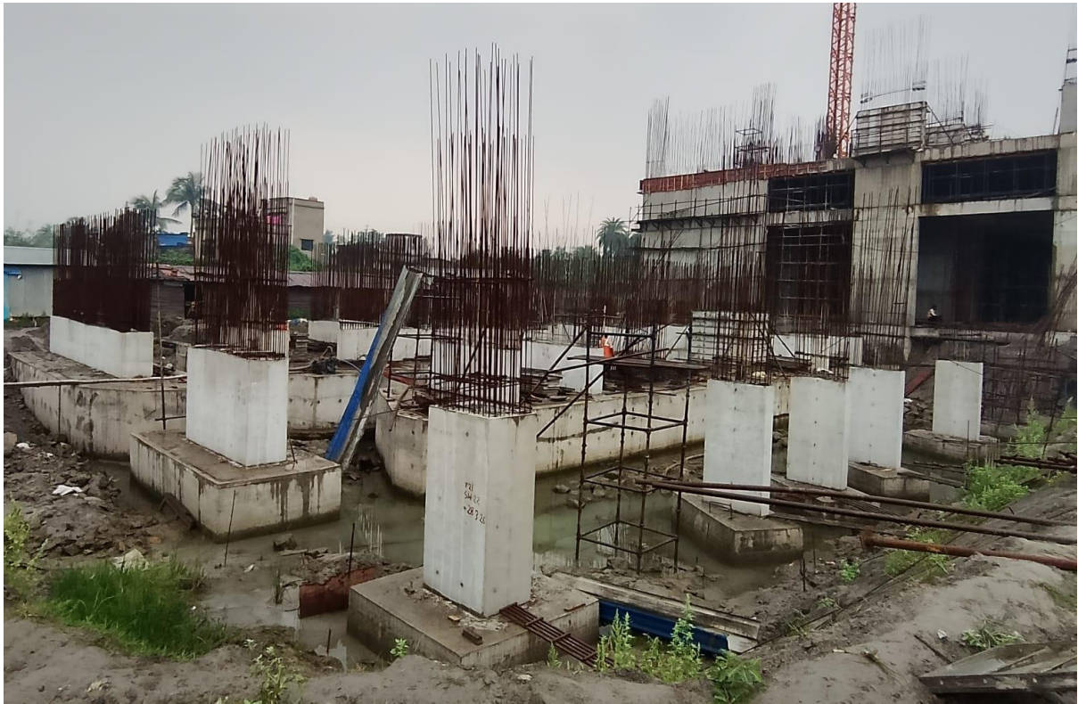
Tower 20- Tie beam shear wall work in progress.
